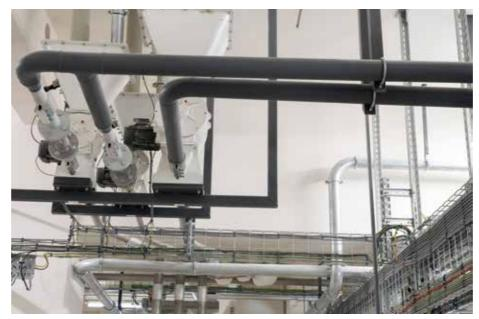
Downstream of every pipe is a blower, some leading from the ground floor to the eighth floor. The grey pipes supply the raw gas. As soon as food is involved, stainless steel tubes are used (silver).
