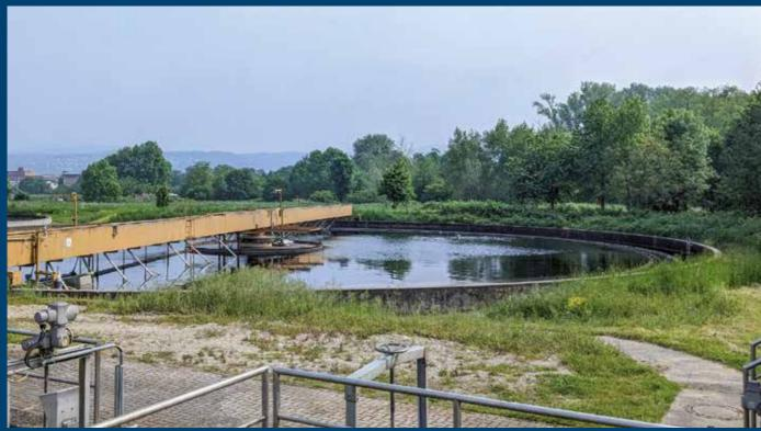
The aeration phase is followed by secondary treatment in the Sinzig wastewater treatment plant in two circular basins.
