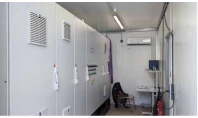
The control system for the turbo blowers is housed in a separate container. As the technology of the wastewater treatment plant was destroyed by the flood, the control of the mobile rental solution runs
