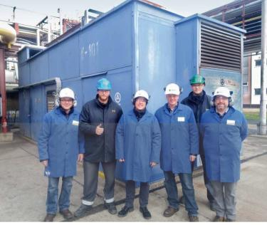
One of several VRa 736SDs for the compression of lime kiln gas with turbine drive - year of construction 2008.
